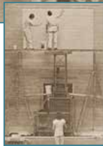
Above: The completed murals were smoothed into place from top down via a method much like wallpapering. Inset: Three workmen from Theodore Lawrence, Inc. began phase one of the mural installation process – coating the blank panels on the west wall with an adhesive.
