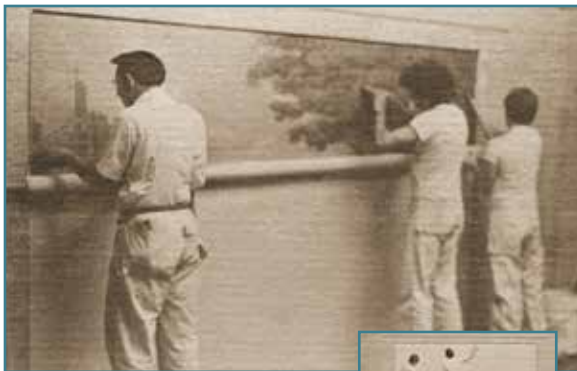
Above: The completed murals were smoothed into place from top down via a method much like wallpapering. Inset: Three workmen from Theodore Lawrence, Inc. began phase one of the mural installation process – coating the blank panels on the west wall with an adhesive.
